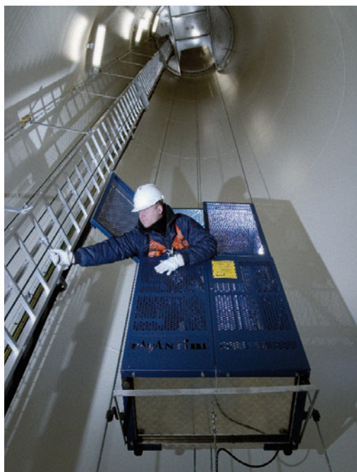
The Avanti Service Lift turns around its own axis and follows the ladder from the bottom to the top of the wind turbine.
