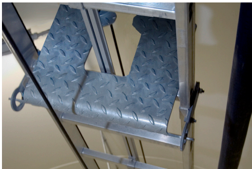
Ladder with rest platform mounted with omega bracket.
