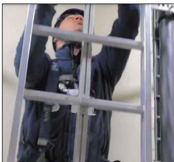
**Step 3** – With a solid body position technician 1 grabs the hanging safety wire with gloved hands. Then holds tight on the safety wire and performs a fast hard lateral heave towards his/her body.
